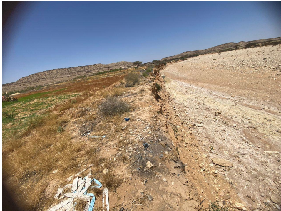
Figures 5 & 6: Observation on Rabaable's stream due to Gully caused by heavy rainfall water.
