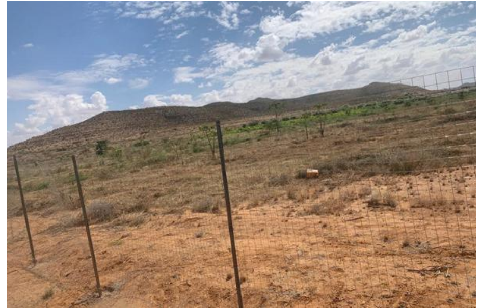
Figure 2: Completed Fencing at Rabaable site.
