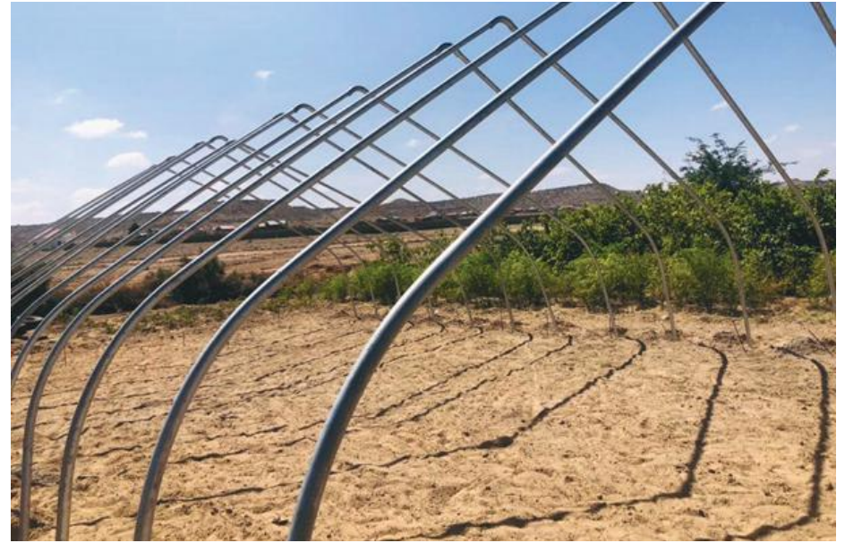
Figure 10: Completed drip irrigation at Balley site.
