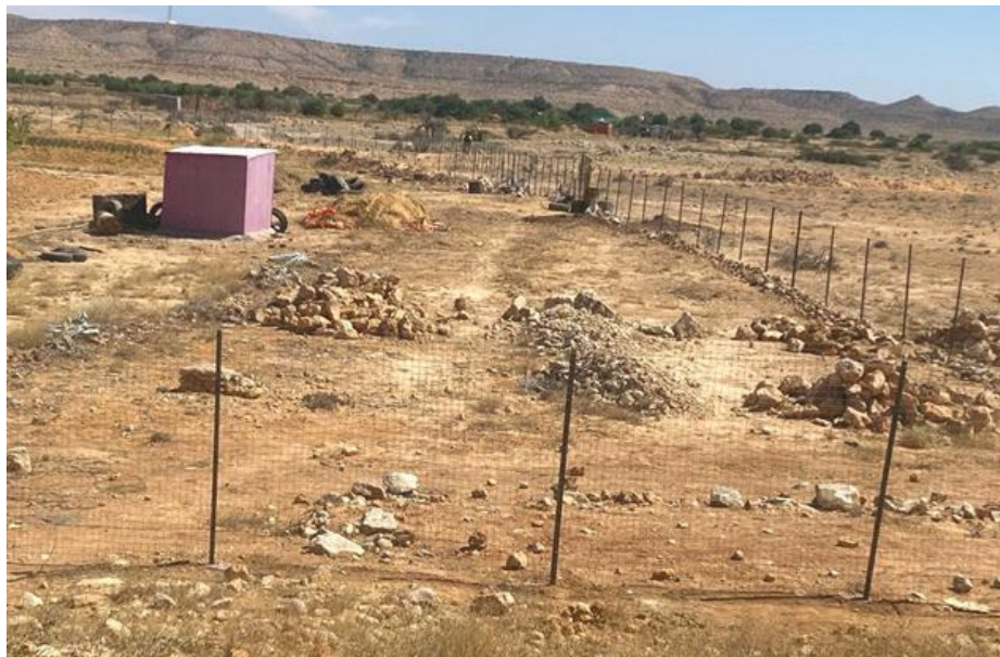
Figure 5: Completed drip irrigation at Cuun site.
