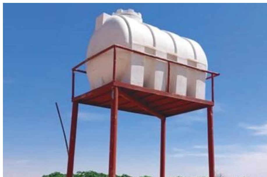
Figure 8: installed water tank at Balley site for efficient use of drip irrigation.
