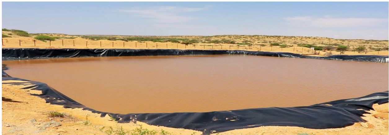
Ilma-dheer Water Catchment after rehabilitation
